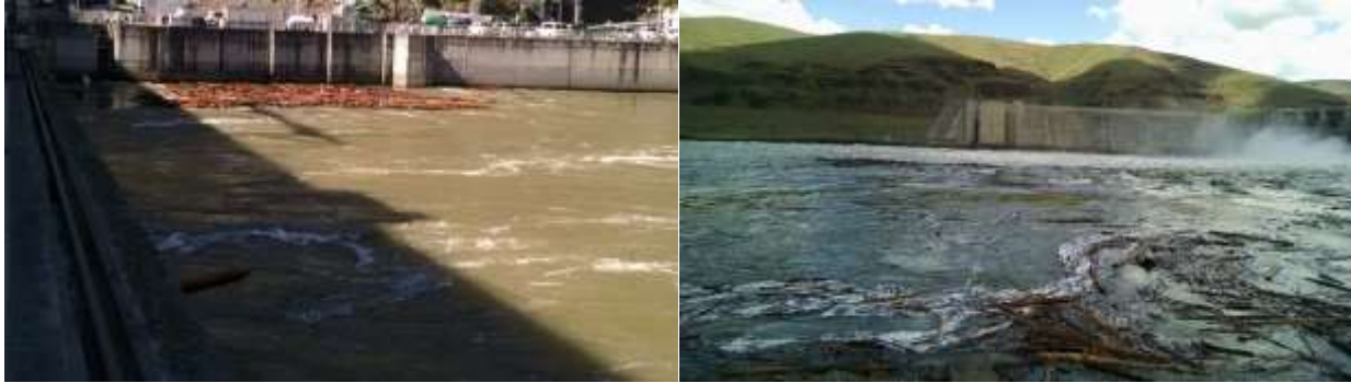
Figure 2. Lower Granite Dam tailrace debris on 15 May 2017.
